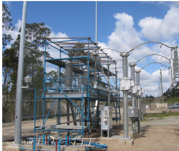
Figure 1: Scaffolding Around 110kV Outdoor Termination
