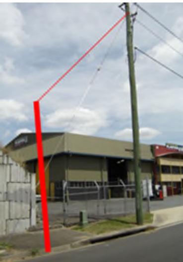
EP36M - Recover stay and install pole stay.
