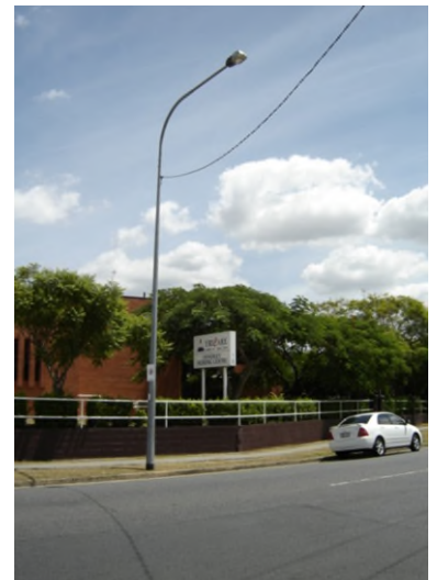
EP38M – Replace single streetlight with an overhead connection.
