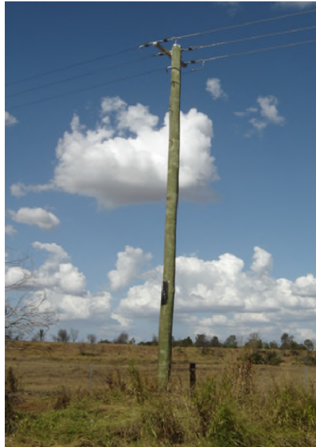
EP10M – Replace 11kV shackle pole
