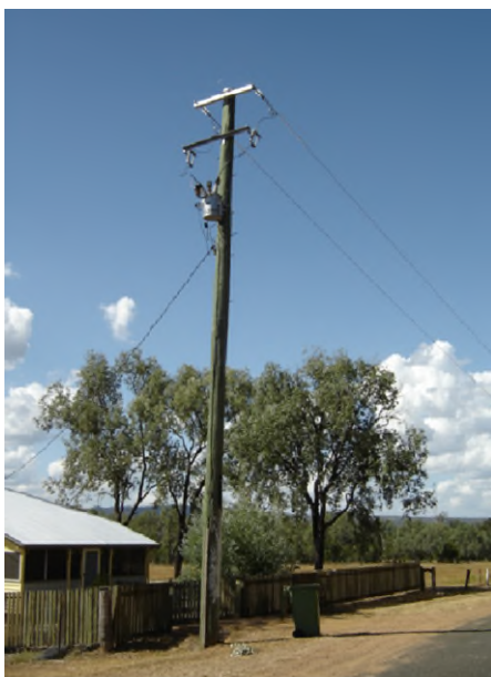
EP12M – Replace 11kV termination pole with single phase transformer
