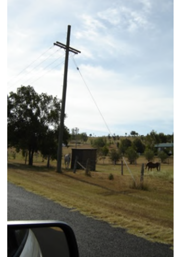
EP35M - Relocate ground stay only.
