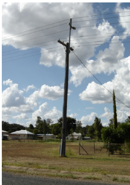
EP13M – Replace LV pole with 11kV riser attached
