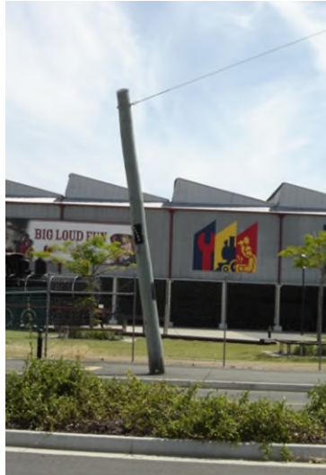
EP34AM – Replace single stay pole
