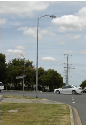
EP37M – Replace single streetlight supplied via an underground cable.
