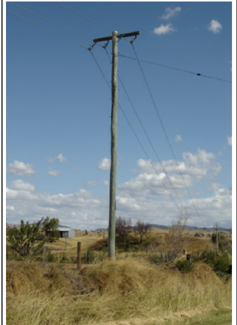
EP11M – Replace 11kV angle pole with head stay attached.
