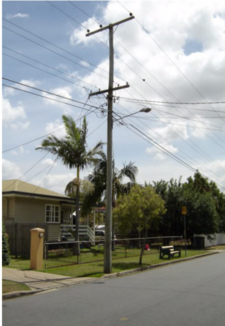
EP9M – Replace 11kV in-line pole in quiet street
