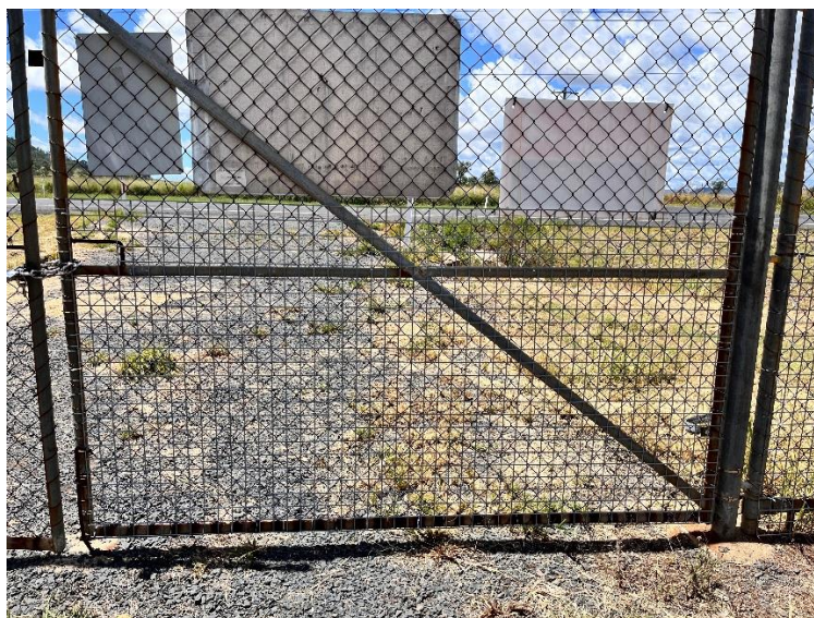
Figure 2 - Secondary fence mesh installed on existing chain link fence
