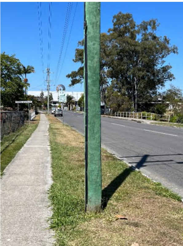
View of base of pole also showing the MEN down conductor on the pole. (Note the sun is behind the camera)
