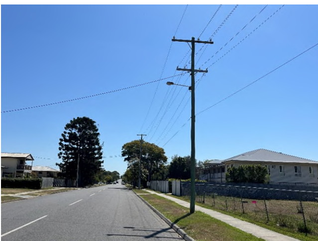
View of the pole looking in the opposite direction along the roadway / street.
