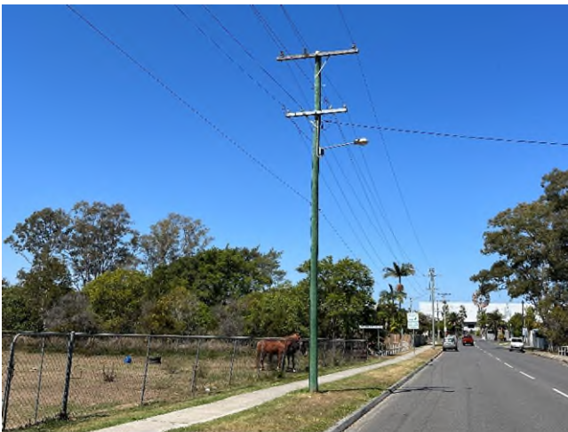
View of the pole looking in one direction along the roadway / street
