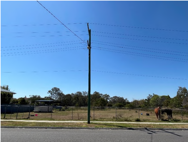
View of the pole from across the roadway / street
