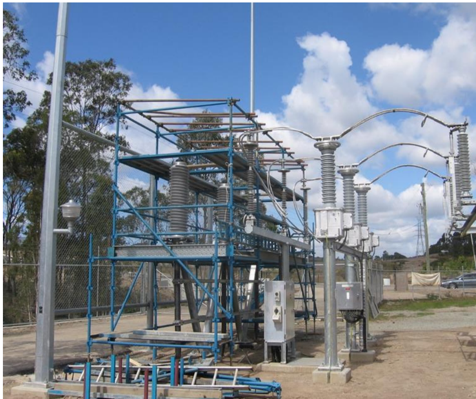
Figure 1: Scaffolding around 110kV outdoor termination
