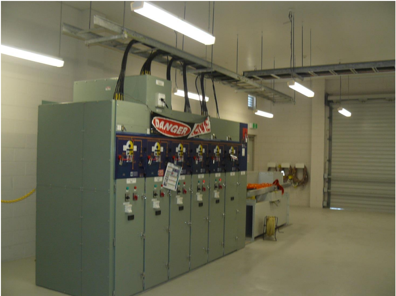
Figure 33: Sample nonwithdrawable switchgear
