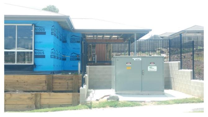
The Energex Underground Distribution Construction Manual (6229-A4) Section C3 Sub-Sect 1 Sheet 1 states that the edge of all Padmounted substation (PMT) enclosures shall be located a minimum of 4m from the edge of a permissible residential dwelling construction area (to address noise, EMF and fire and explosion risk).
